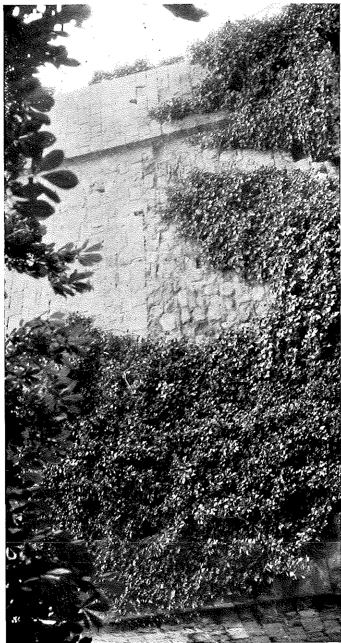
FIG. 2.—LOWER PART OF TOWER, FROM THE NORTH. Norman masonry is evident in the buttresses and in the facing of the upper part; the original wall is seen below, between the buttresses.
