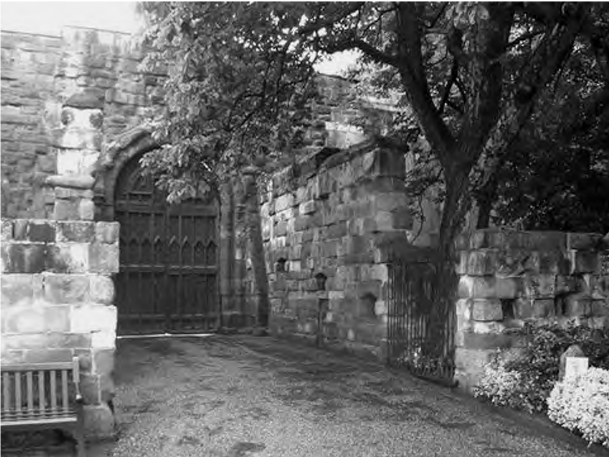
Plate 2 Shrewsbury Castle, the remains of the stone-built barbican/gate house completed in February 1644. Built by the Royalists to defend the Castle's otherwise vulnerable main gate, the loopholes in the passage would allow muskets, and possibly light cannon, to enfilade the adjacent curtain wall. (Author's photograph)
