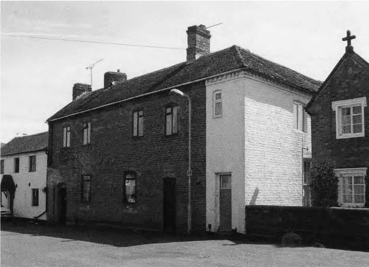
Plate 6 Newport. The former Newport parish workhouse (pre-1787) in Workhouse Lane (now Vineyard Road).
