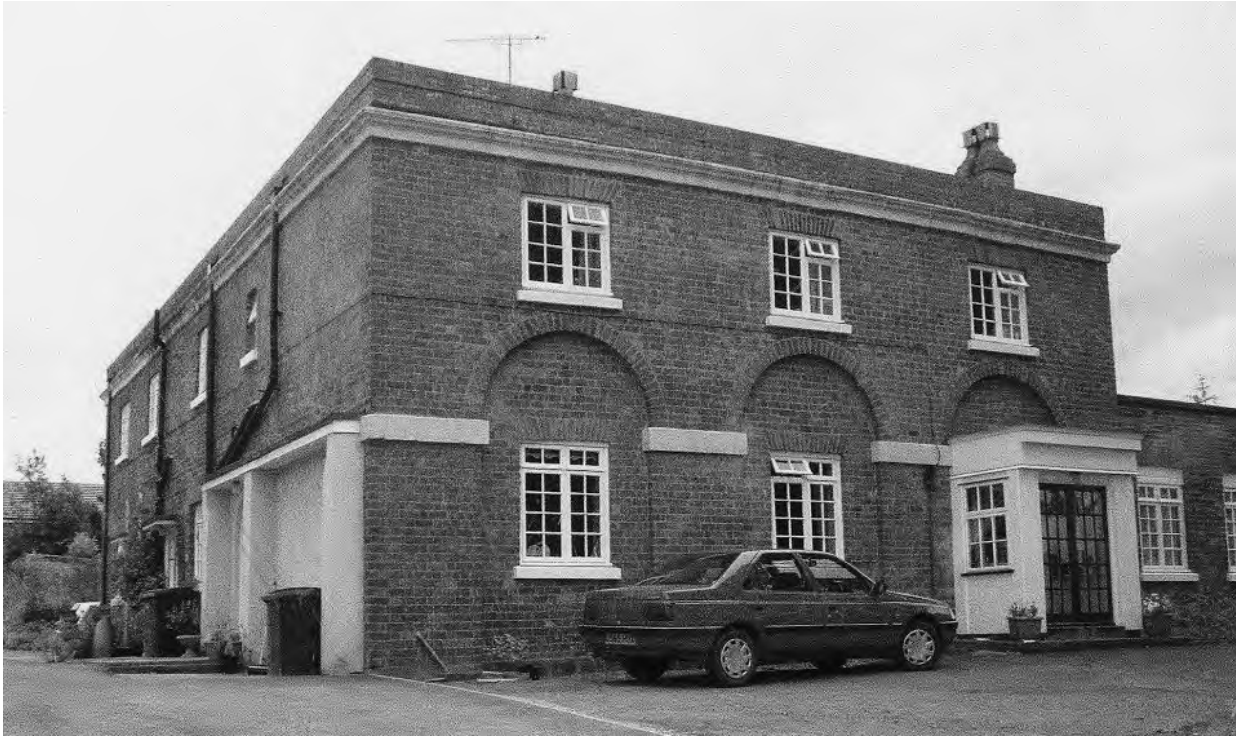
Plate 3 Oswestry. The surviving west front annexe of the former house of industry at Morda. It was joined to the main building by a single storey link at the left of the near corner. This annexe was known later as the Nightingale Wing and is now called Morda Court.
