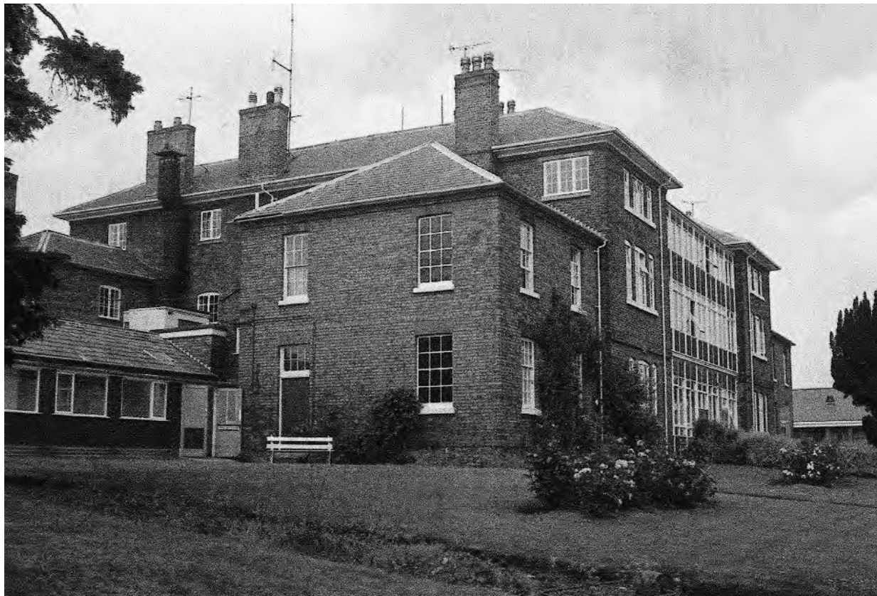
Plate 4 Whitchurch house of industry as altered to Deermoss Hospital in the mid-20th century. View of original from south. (Permission of Shropshire Archives: PH/W/18/7.)
