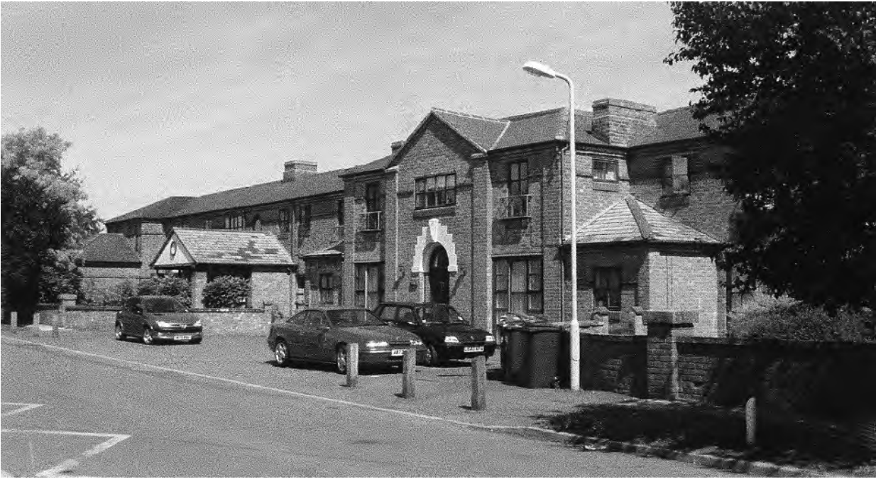
Plate 7 Newport. The former Newport union workhouse of 1855–6 in Audley Avenue (now known as Audley House).
