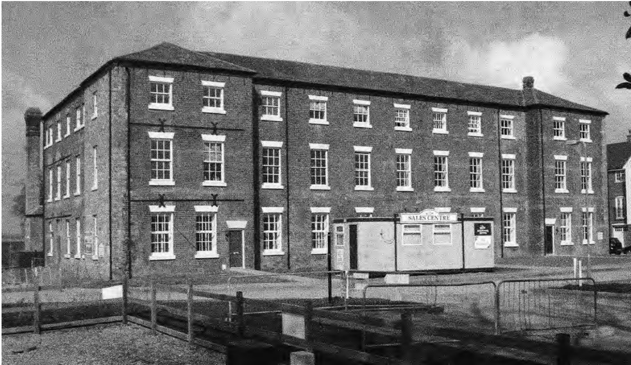
Plate 2 Atcham. The former house of industry (later Berrington Hospital) at Crosshouses, following demolition of the wings at left and right and conversion into dwelling units (2005). The chimney at rear belonged to a laundry in the former infirmary building.
