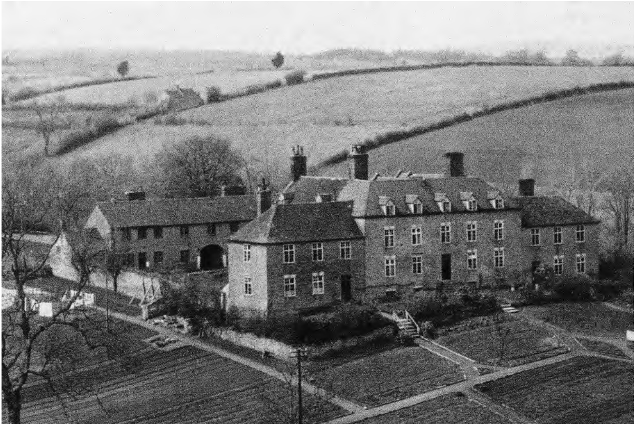
Plate 14 Cleobury Mortimer. The workhouse in the late 19th century or early 20th century. (Now demolished.) The central part is the original parish workhouse. It was considerably enlarged in the 1830s and 1840s. (Permission of Shropshire Archives: PH/C/23/2(B).)
