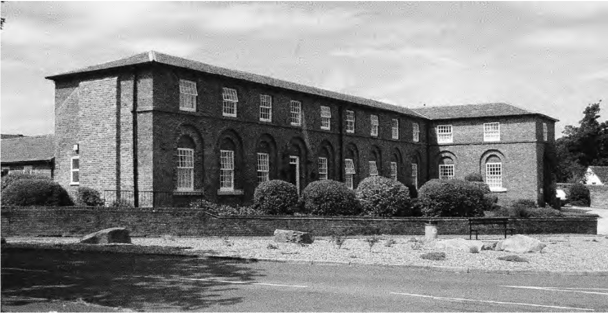
Plate 8 Shifnal. The former Shifnal parish workhouse, 1817, enlarged to serve as Shifnal union workhouse after 1836.
