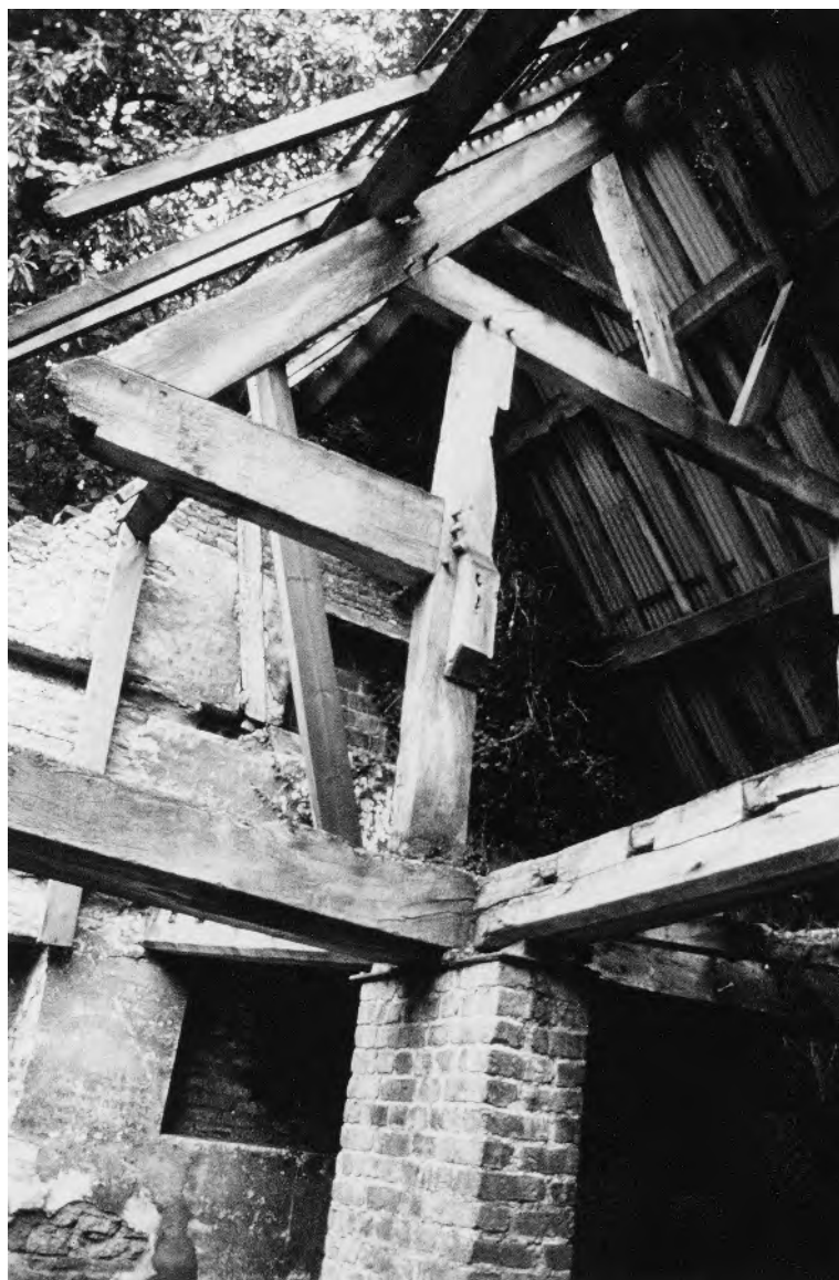
Plate XIII Madeley Court barn: roof and attic floor frame of south-west wing, including Truss 11, prior to collapse (Bob Meeson).
