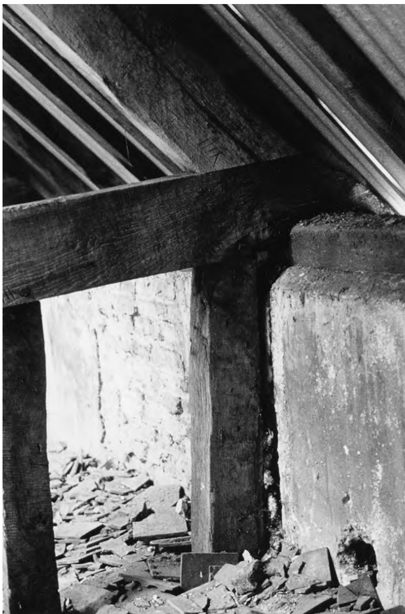
Plate XII Madeley Court barn: detail of roof frame of north wing prior to collapse showing truss and wall-plate assembly with a carpenter's number on principal rafter.
