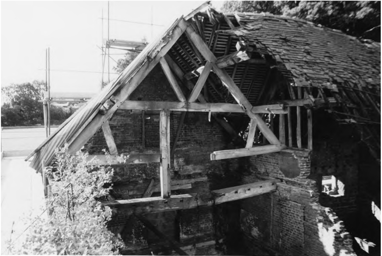
Plate VIII Madeley Court barn: Truss 2 prior to removal.
