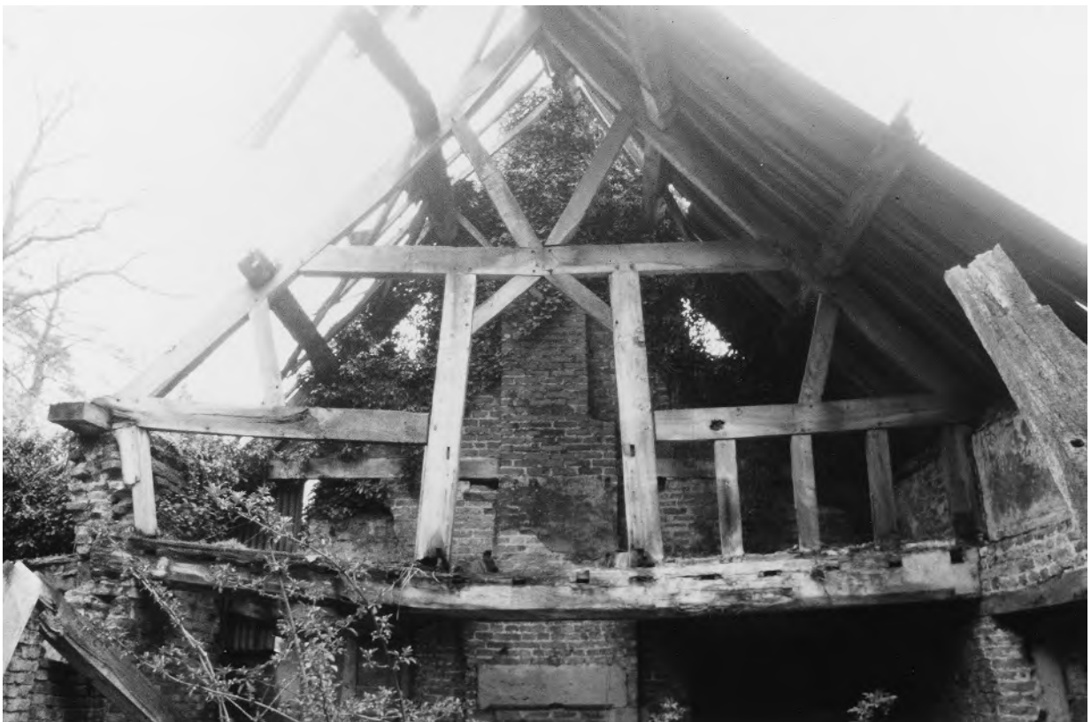
Plate IX Madeley Court barn: Truss 8 prior to removal.
