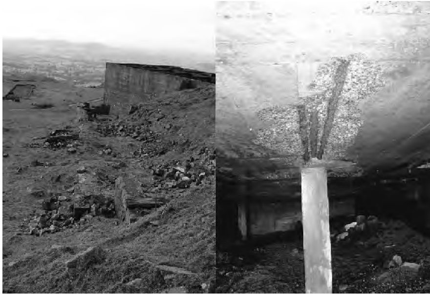
Figure 5: Left: Ferro-concrete hopper (background) and incline plane engine house (foreground); Right: Eroding support beneath ferro-concrete hopper. Photos: Glynn Barratt.
