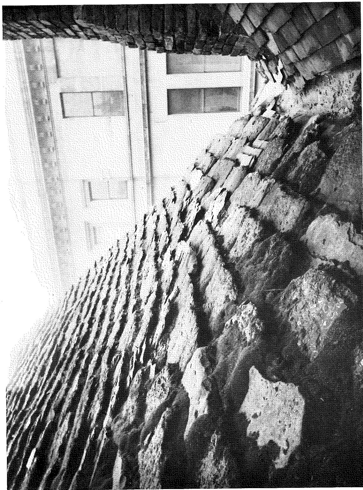
FIG. 1 HARNAGE SLATES ON LLOYD'S MANSION, SHREWSBURY, 1985 (LOCAL STUDIES LIBRARY, SHREWSBURY) 1895
