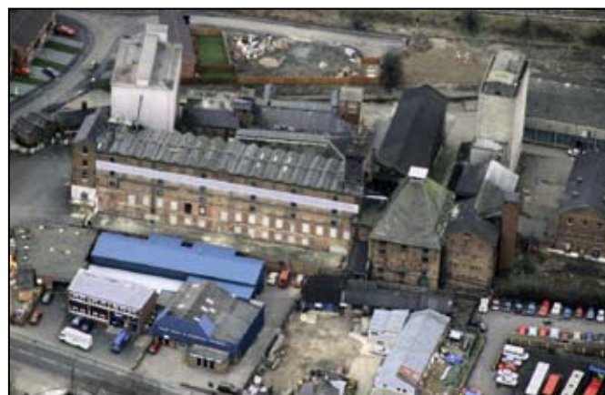
Ditherington Flaxmill Maltings from the air in 1995 (©CPAT 95/C/1530 21/03/1995)
